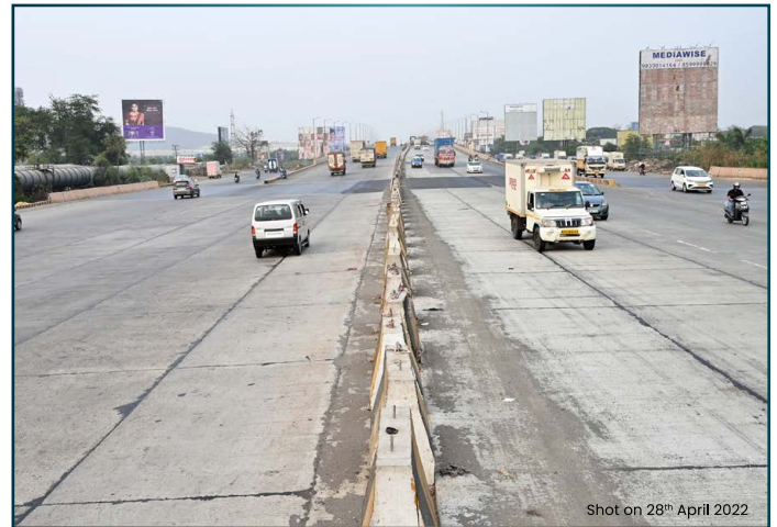
Ready Rajnouli over-bridge
