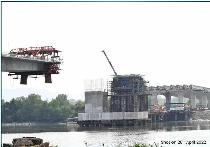
Under construction Dombivali-Mankoli bridge
