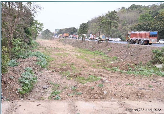
Widening of Mumbai-Nashik Expressway
