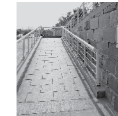
Ramps provided at all entrance areas to improve accessibility for differently abled and wheelchair users
