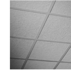
Toilets designed with under deck plumbing design and provided with grid false ceiling for easy maintenance or repair
