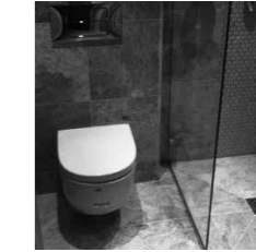
Toilets strictly designed to divide dry and wet areas. Shower area provided with a step down of 1-1.5 inches to avoid water spilling over to the dry area
