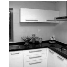
Kitchen granite platform placed at height of 825 mm taking into consideration the average height of Indian Women
