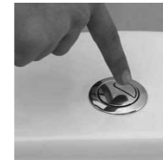
Water conservation in toilets by fitting them with two button flush tanks designed for light and heavy usage
