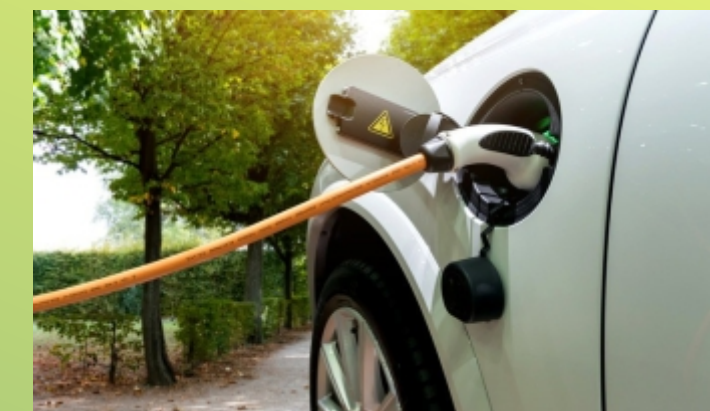
Electrical Vehicles Charging Bay
