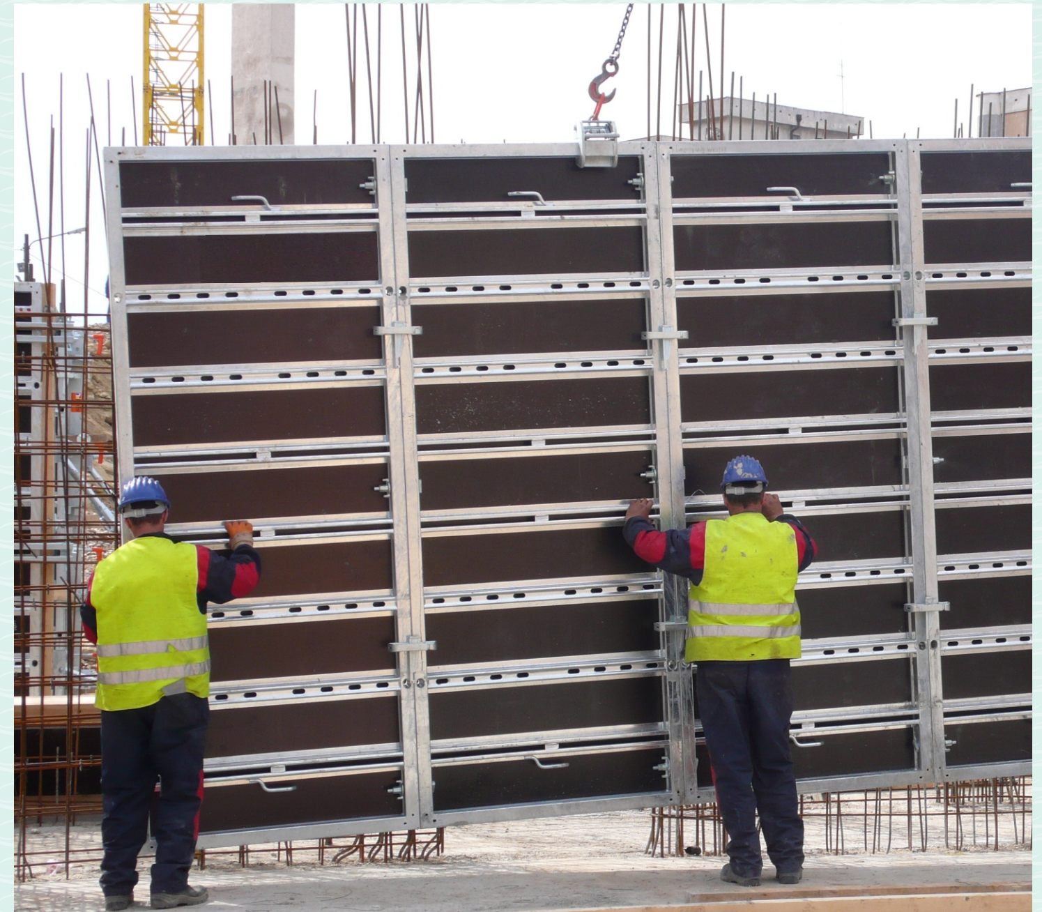
Tower A / Tower B / Tower C / Tower D: Construction Technology used – System Aluminium Formwork Tower E: Construction Technology used – Conventional
