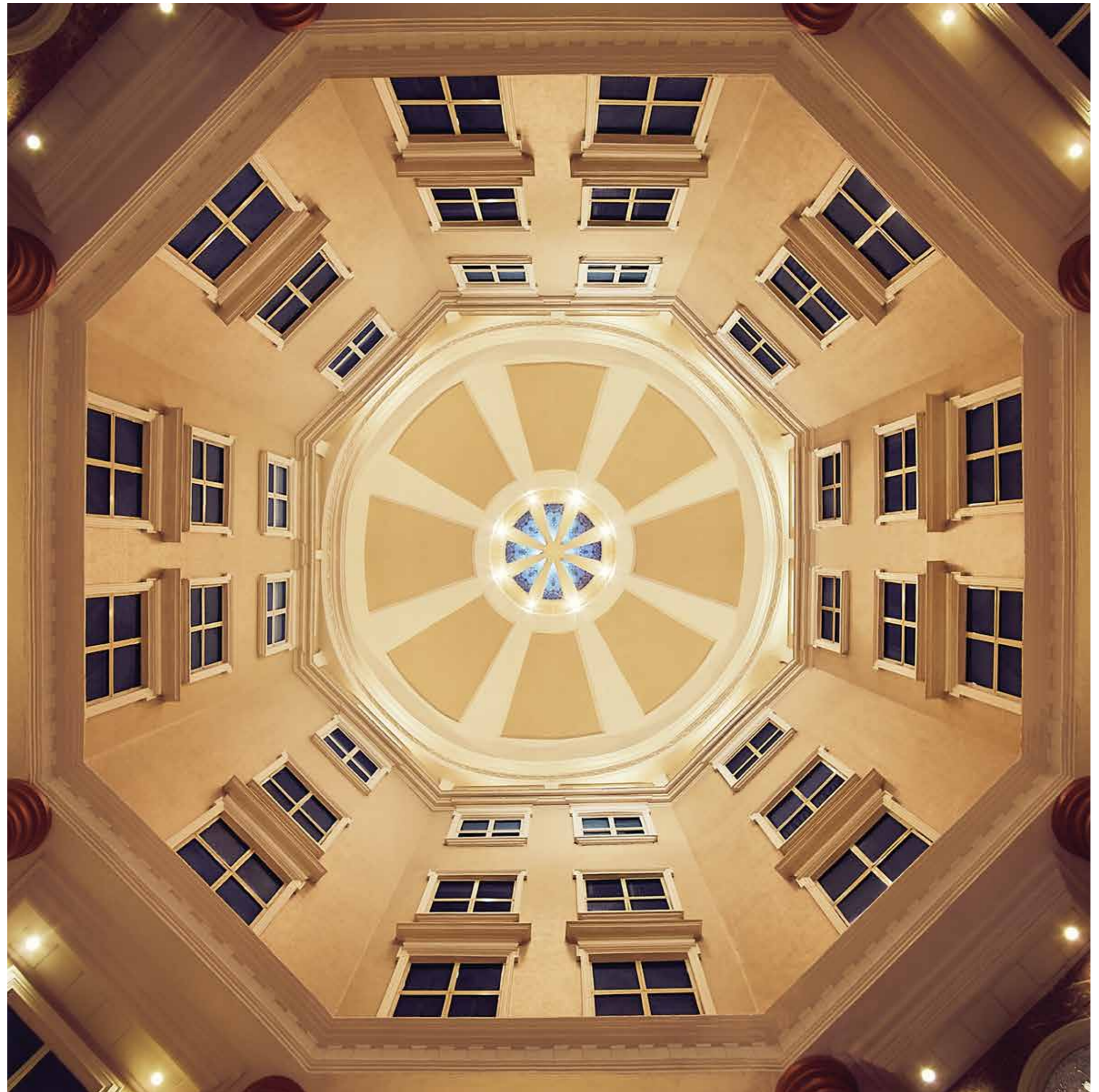
Interior image of Olympia, Hiranandani Gardens, Powai.
