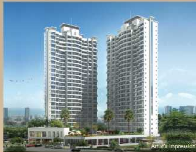
REGENCY CREST KHARGHAR, NAVI MUMBAI
