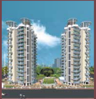
ACTUAL PHOTOGRAPH SAI PEARLS KHARGHAR G+15 Storeyed 2 Towers
