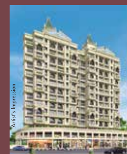
ACTUAL PHOTOGRAPH SAI FORTUNE ULWE G+13 Storeyed Tower
