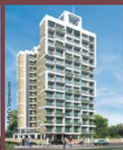
ACTUAL PHOTOGRAPH SAI GANGA ULWE G+13 Storeyed Tower
