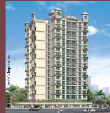
ACTUAL PHOTOGRAPH SAI JEWEL KHARGHAR G+18 Storeyed Tower
