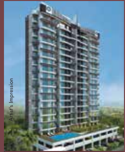
ACTUAL PHOTOGRAPH SAI WONDER KHARGHAR G+18 Storeyed Tower
