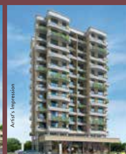
ACTUAL PHOTOGRAPH SAI SAHIL ULWE G+12 Storeyed Tower
