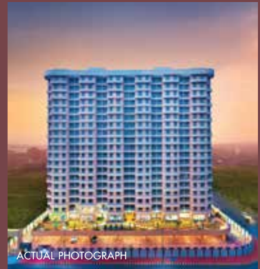
ACTUAL PHOTOGRAPH SAI RIVERDALE TALOJA G+19 Storeyed Tower with 2 Wings
