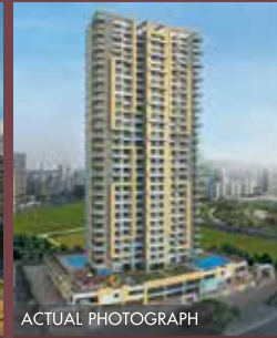
ACTUAL PHOTOGRAPH SAI SOLITAIRE KHARGHAR G+30 Storeyed Tower
