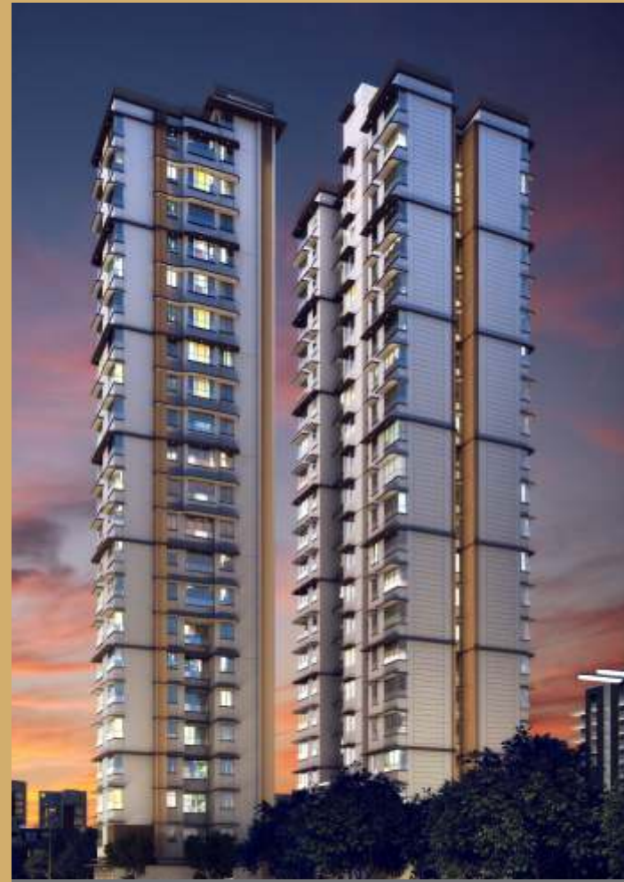
Unity Towers - Worli
