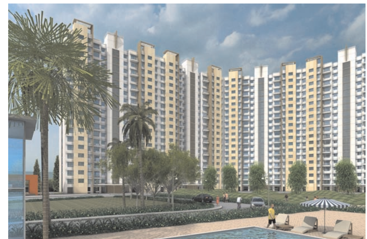
3 BHK TOWERS - CLUBHOUSE SIDE
