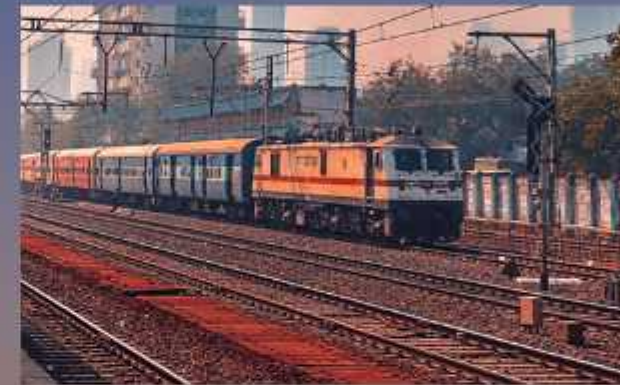
Upcoming Dedicated Freight Corridor passing through Vasai will promote economic growth and development in the area
