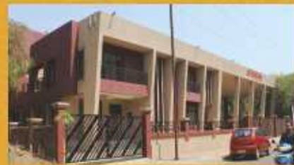
FIRE STATION - KOPERKHAIRANE
