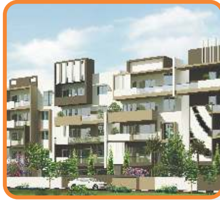
VRR Stone Arch Hennur Main Road
