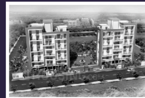
Fortune Mirador Baner, Pune
