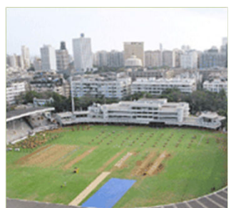
Brabourne Stadium, Mumbai
