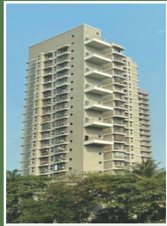
BLDG NO.14 - KANNAMWAR NAGAR
