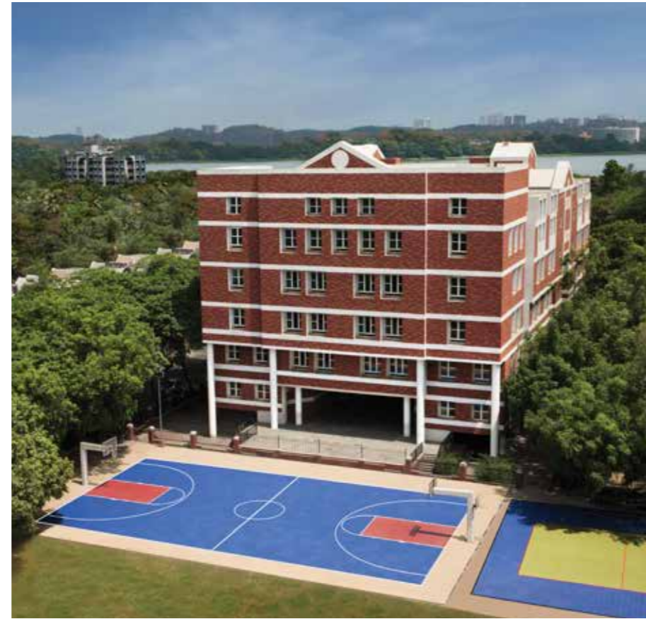
ACTUAL IMAGE OF HIRANANDANI FOUNDATION SCHOOL
