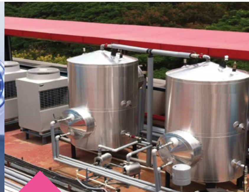
Centralised heat pumps and solar power that provide hot water directly to your taps, helping you cut energy consumption. It's time to bid farewell to bulky old geysers.
