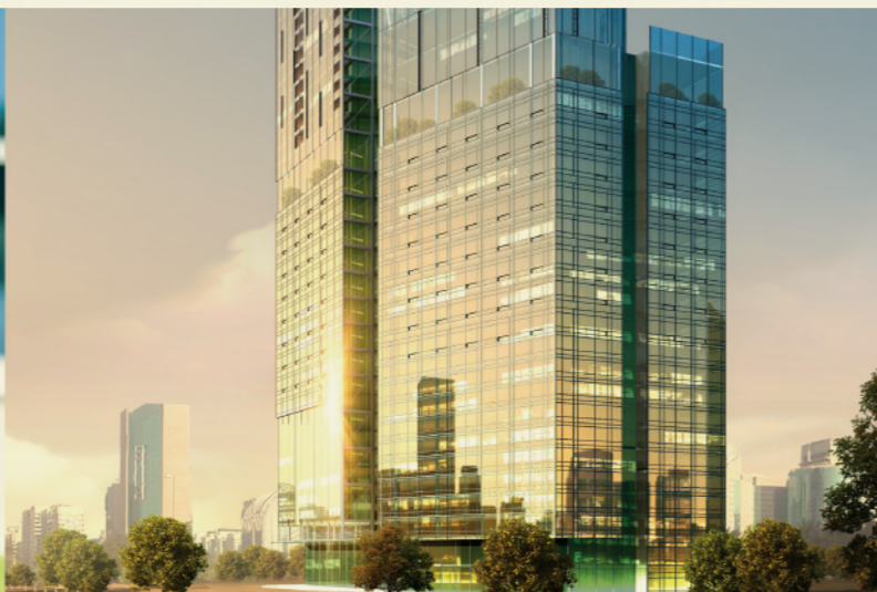
Next to MNC Offices
