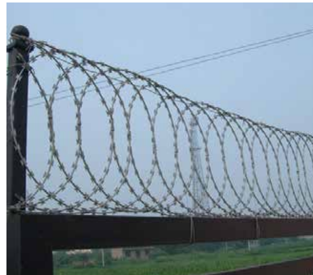
Walled perimeter wired with adequate anti-scaling measures
