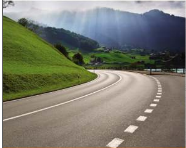
Development of Roads, Water Supply & Civic Services by Panvel Municipal Corporation
