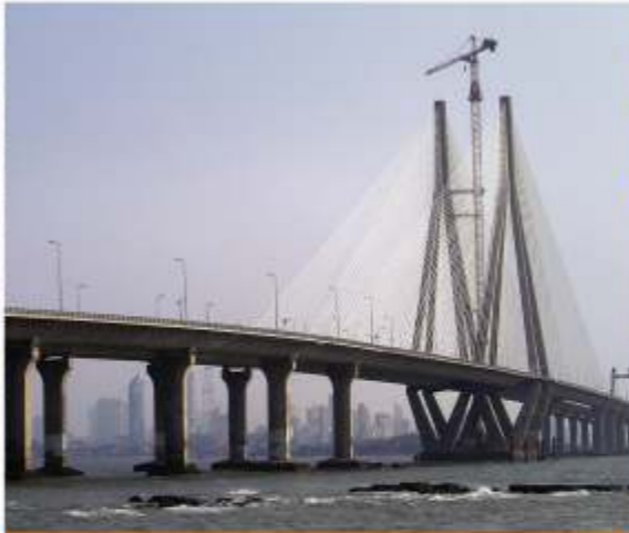
Hon. Prime Minister Laid the Foundation Stone (Dec.2016) of Mumbai Trans Harbour Link
