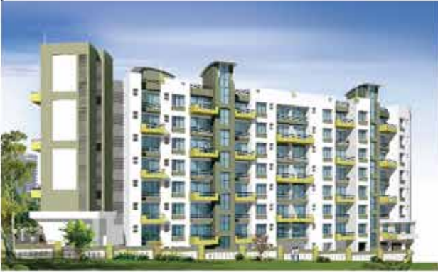
Shreenathji Tower, Kalyan west
