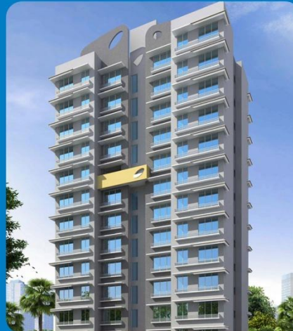
HIRAL LEGACY ONGOING PROJECT, KANDIVALI
