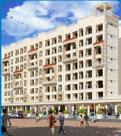
HIRAL SHREE SAMARTH PAST PROJECT, MIRAR ROAD
