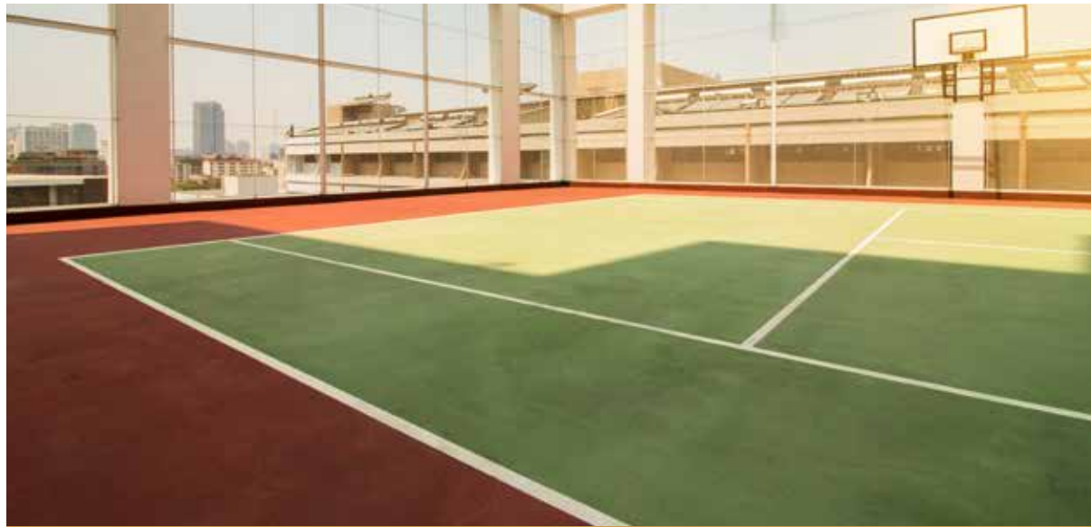
Rooftop LED Multipurpose Court
