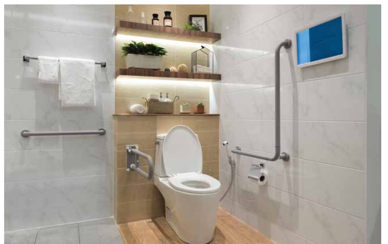
HAND RAILING IN ONE TOILET
