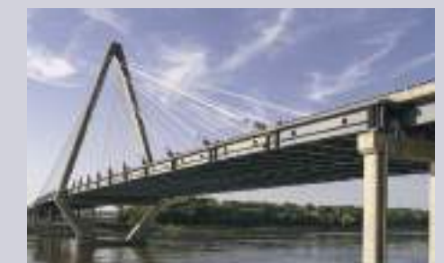
2 new bridges over Thane creek speeding up Mumbai- Nashik travel
