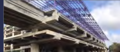
Kadugodi Metro Station
