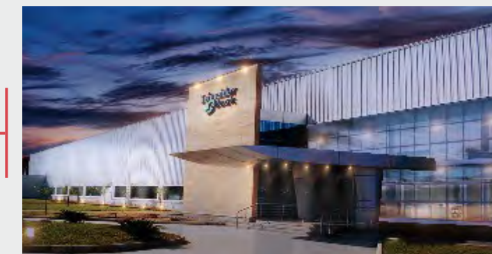
SCHNEIDER ELECTRIC Hyderabad, Telangana
