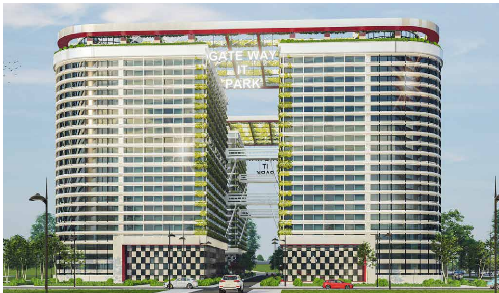
Gate Way IT Park, Kandlakoya
