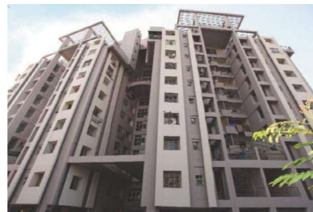
Merlin Regency, Suresh Sarkar Road - Entally
