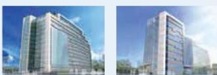
MAGNUM TOWERS (I & II) Sec - 58, Golf Course Extn. , Gurugram
