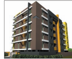
Madhavi Towers Rambagh, Attapur
