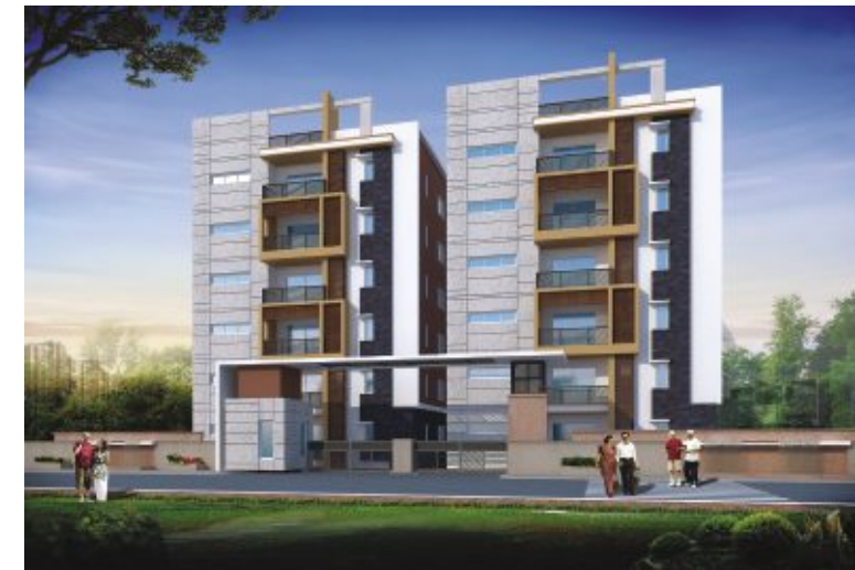
Lansum Madhav Towers, Madhapur, Hyderabad
