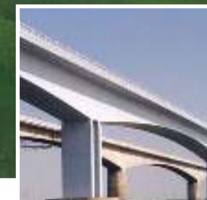
NAIGAON E/W BRIDGE
