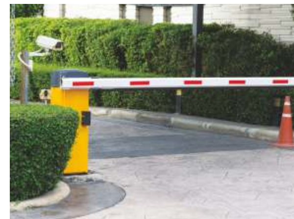
AUTO-CONTROLLED ENTRY & EXIT
