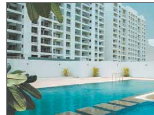
GODREJ HORIZON NIBM ANNEX, PUNE Completed in 2015
