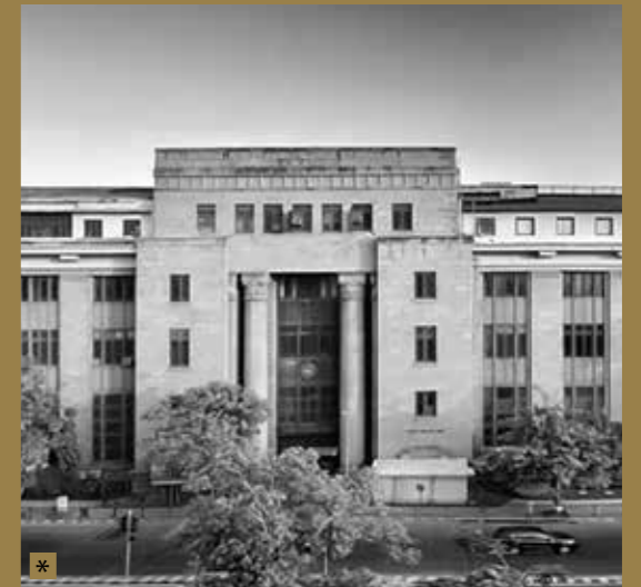
RESERVE BANK OF INDIA BUILDING, MUMBAI
