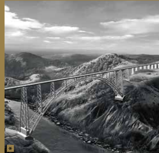
CHENAB RAIL BRIDGE
