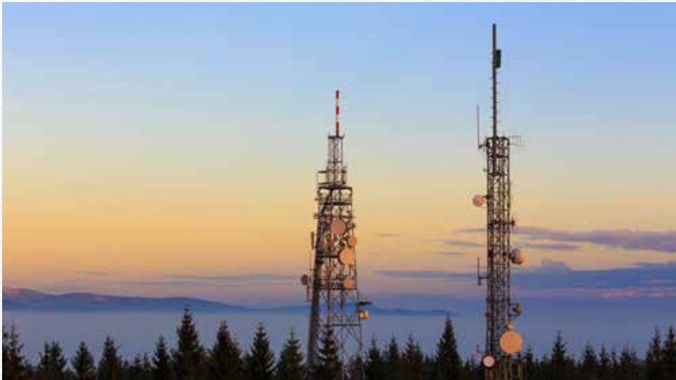
ELECTRICAL & COMMUNICATION NETWORK PROVISION
