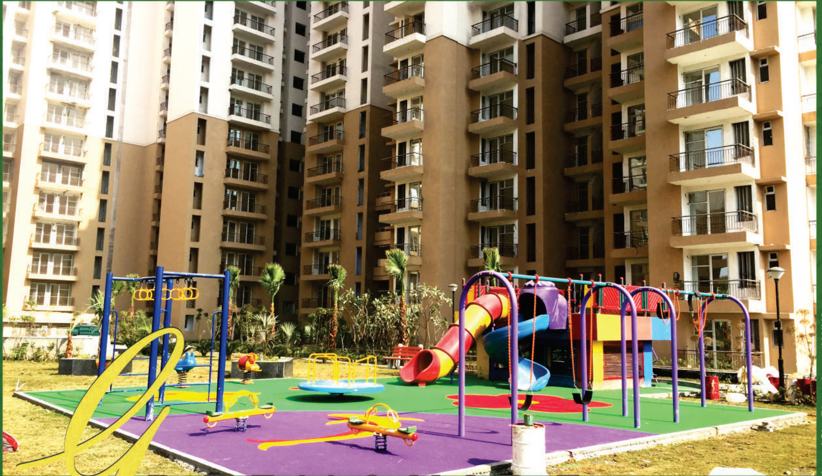
Actual Site Photo As on JAN'18
