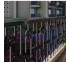
RAILING WROUGHT IRON RAILING
