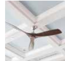
CEILING OIL BOUND DISTEMPER
