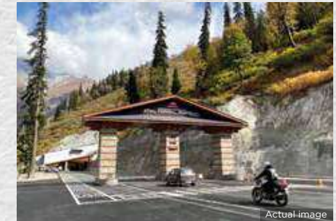
Atal Tunnel, Himachal Pradesh, 2020
