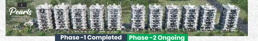
Phase-1 Completed Phase-2 Ongoing
