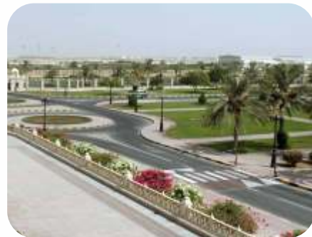
Internal Concrete Road
