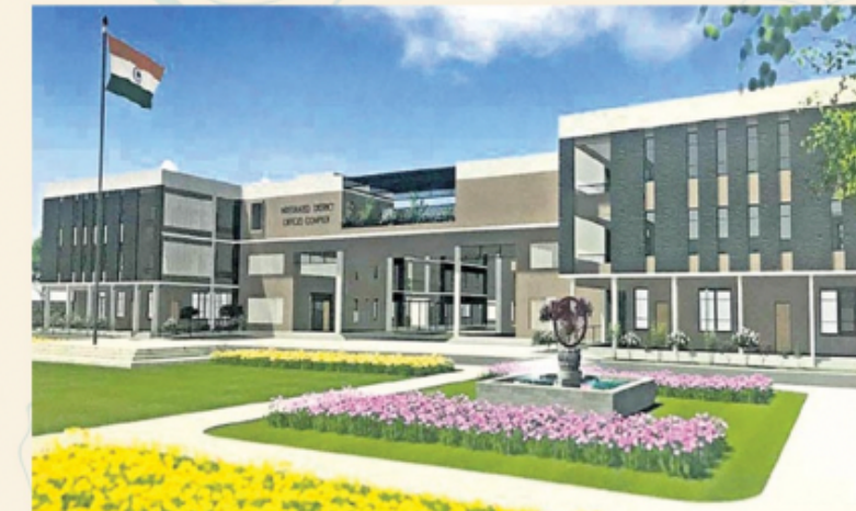
Ranga Reddy Dist Collectorate Office
