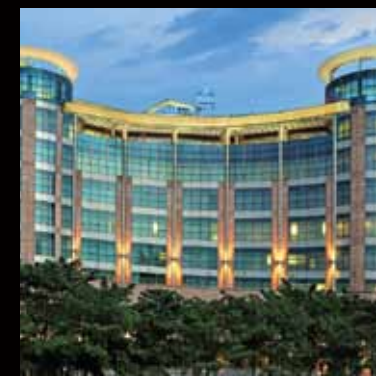
SHALIMAR TCS BUILDING
