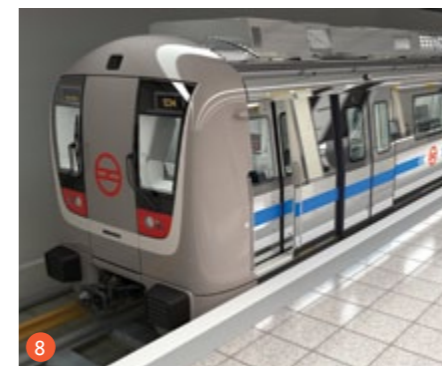
Noida City Center Metro Station
