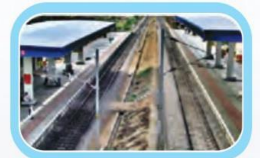
HITEC City Railway Station
