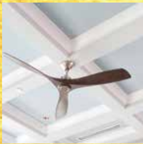
CEILING OIL BOUND DISTEMPER
