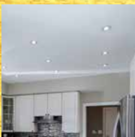
WALL / CEILING OIL BOUND DISTEMPER
