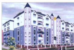
RESIDENTIAL APARTMENTS KONDAPUR
