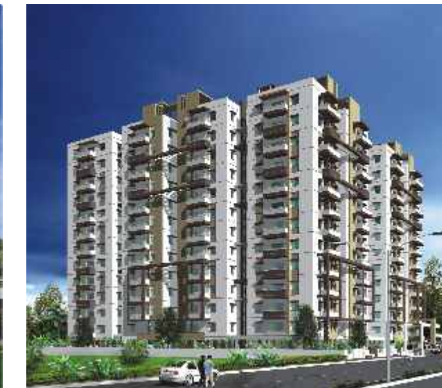
THE RETREAT PROJECT AT KOKAPET IN PROGRESS
