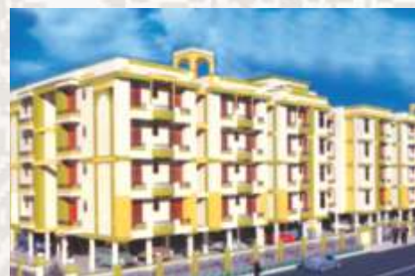
Rudra Apartments Shivpur, Varanasi
