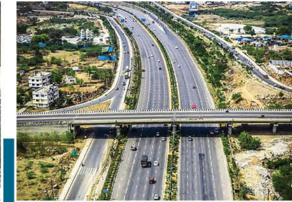
6 Lane Nagpur Highway - NH 44
