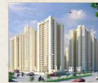
ATS ADVANTAGE PHASE II Indirapuram
